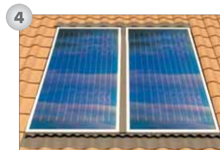
4) Replacement of the exceeding cover removed and final finishing.
